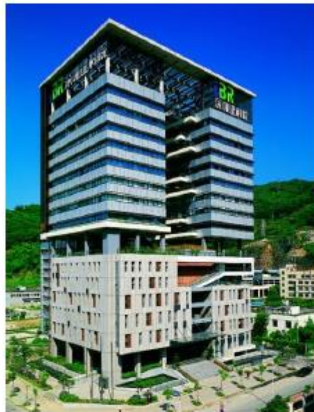
Fig. 2 The iBR building as viewed from the southeast facade
